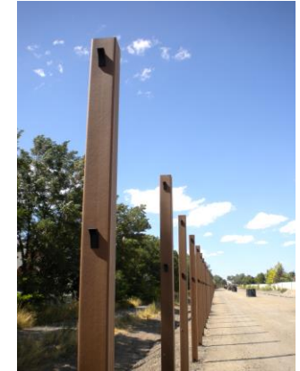
Attach Brackets to Composite Posts at Rail Points
