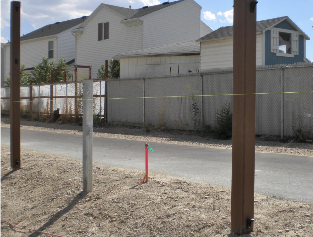
Setting Steel Post Stiffeners and Trex® Composite Post Sleeves
