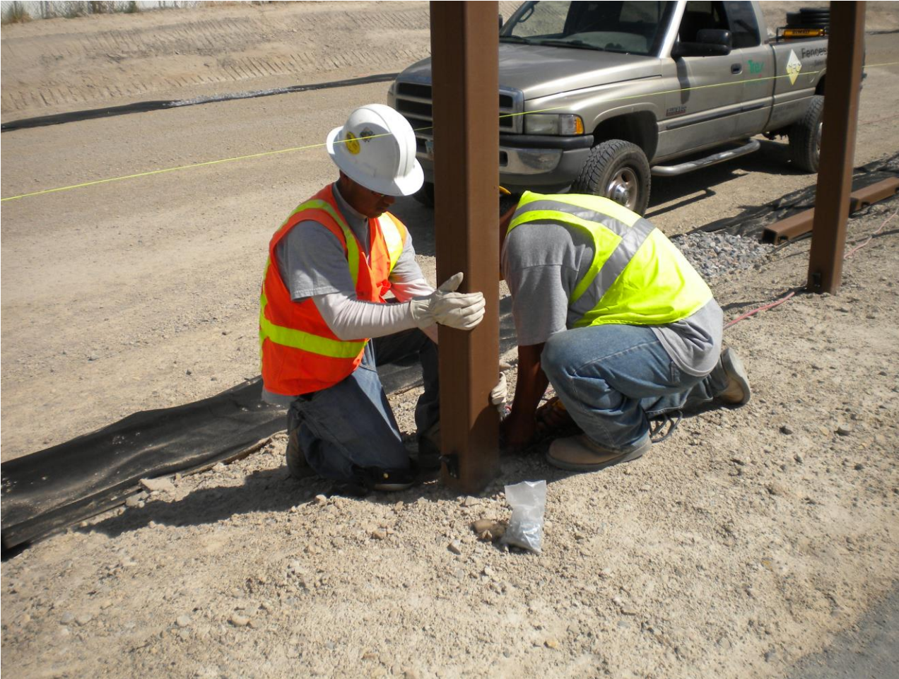
Attaching Fence Brackets
