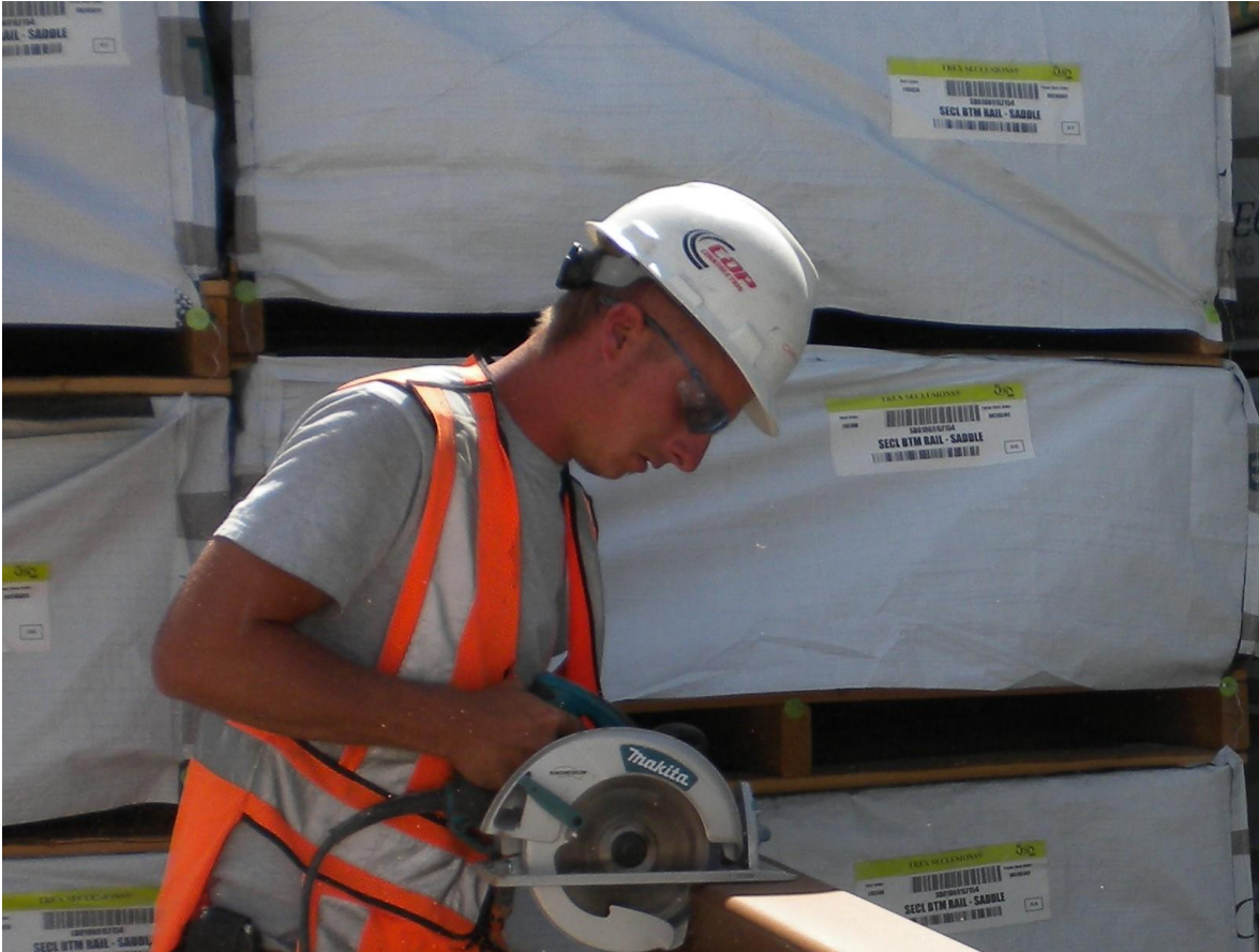
Cutting Rails and Pickets
