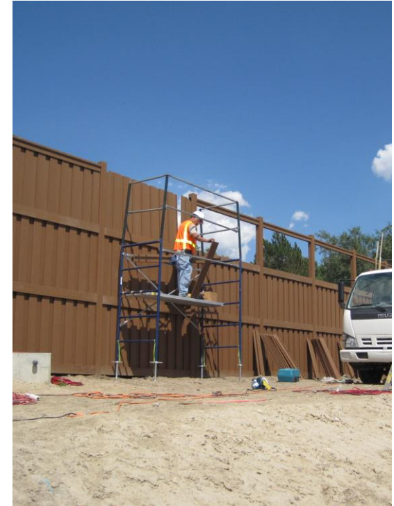
Interlock pickets; place top rail over pickets to ensure fence is secure
